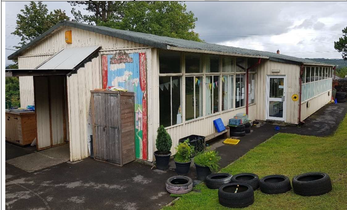
External view of the metal prefabricated building
